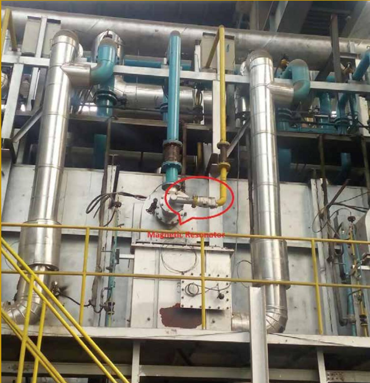
At L&T's Special Steels and Heavy Forgings unit in Hazira, the forging re-heating furnaces are known to be fuel guzzlers. The two furnaces RH-250 and RH-300 account for almost 40% of the total gas used. On-going attempts to enhance efficiency included changing a few operating parameters, reducing leakage through specific maintenance and clubbing of jobs for simultaneous heating, etc. Then came Magnetic Resonators.
