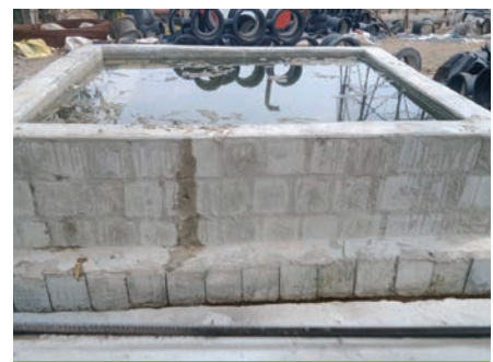
Concrete waste reused for water storage tank
