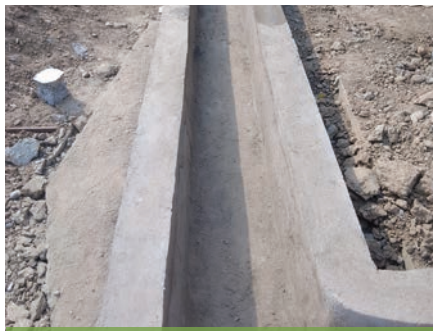
Concrete waste reused to create drains
